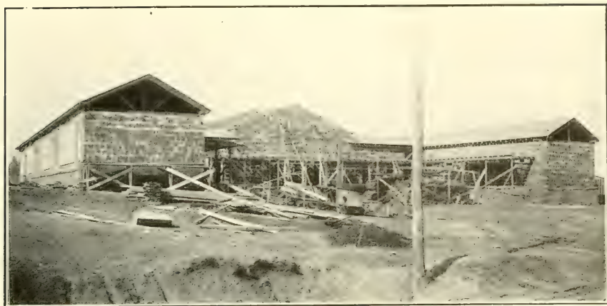
IRVING PARK—GUILFORD COUNTY—SHOWING TILE AND BRICK CONSTRUCTION
